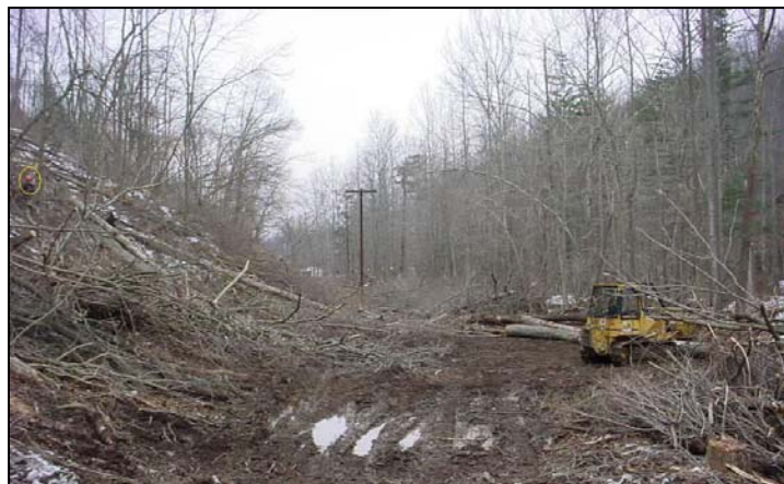
PHOTO 14: Lewis County, KY ~ Bulldozer Clearing R/W
