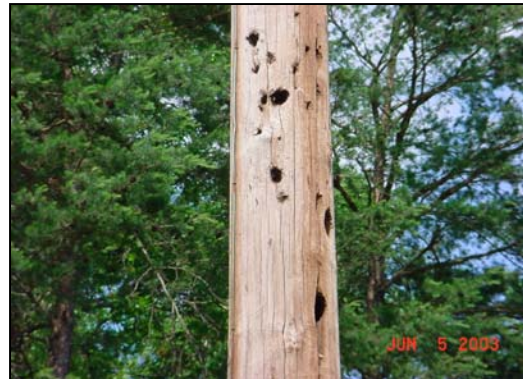
PHOTO 33: Wood Pecker Holes Limit the Strength and Shorten the Life of Wood Poles
