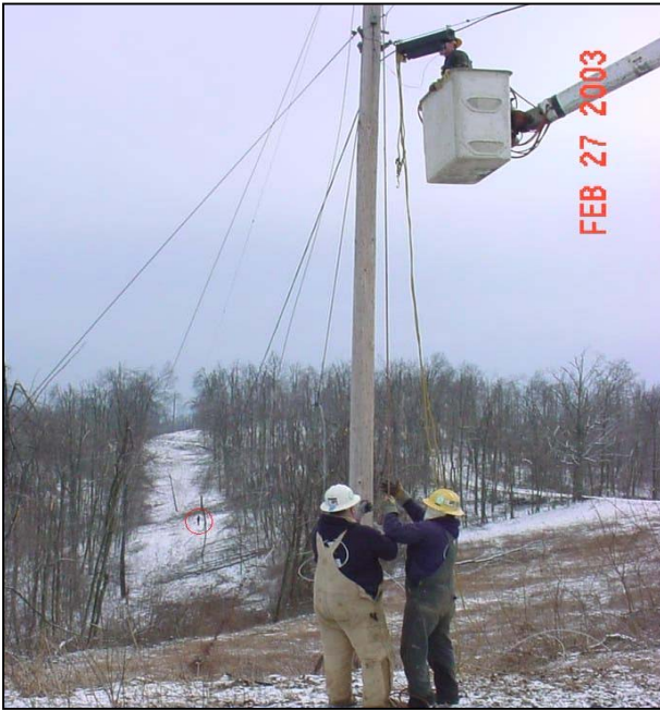
PHOTO 13: Lewis County, KY ~ Pike Contractor and Grayson Crew... Note Lineman in Distant R/W
